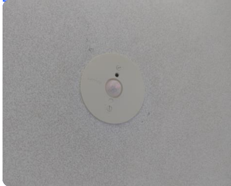
Motion Control Sensor for Wash Room Lighting
