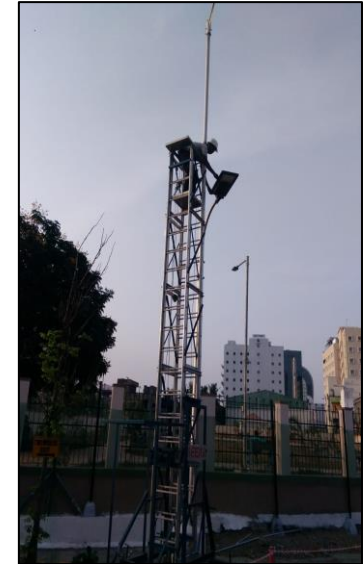
Pole Height is 12 Meters
