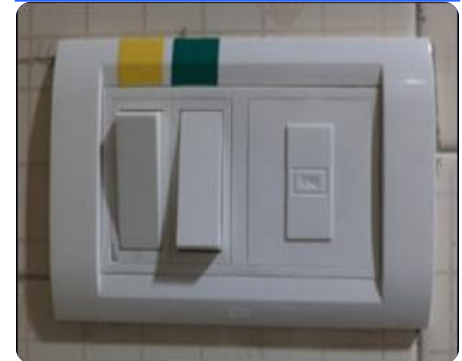
Lighting Circuit Modification with Switch Color Code
