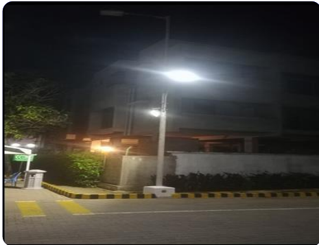
Peripheral light retrofit (250W MHL to 100W LED)
